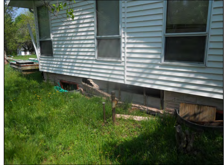
Photograph 2: UST vent and fill lines at Building 57 at Breezy Corners, east-adjacent to the project site.
